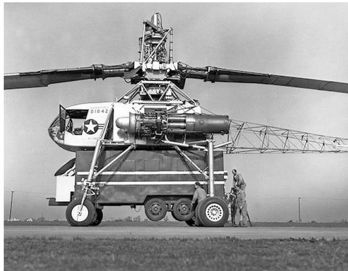
Figure 1 Technicians attach a military communications trailer, weighing 8,000 lbs., beneath the XH-17 to demonstrate the helicopter's immense lifting capability. (Photo from the Ray Prouty collection)
